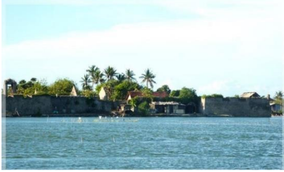
Existing situation of Dutch Fort in Mannar
